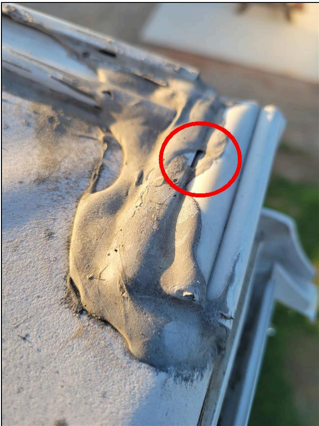
rear cap joint seal - streetside corner
